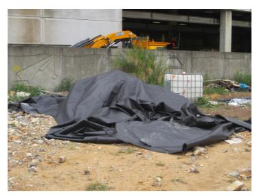
*Photo 1 – Impermeable sheets were observed to have been placed on the stockpiles of excavated soils and rocks that were not in use.*
